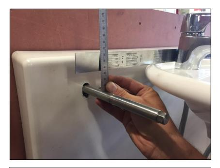
Turn washbasin in against the cover. Place if possible a spirit level onto washbasin. For fitting of fixation of Dock-in to be fastened in correct height loosen fittings a little & adjust them to leave approx. 33mm between fittings & spirit level. Afterwards fasten fittings thoroughly with a spanner.
