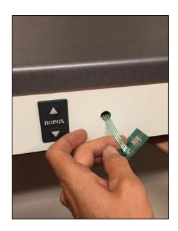
If necessary, put a piece of paint tape on front fascia, to have a guideline for placement of switch.
